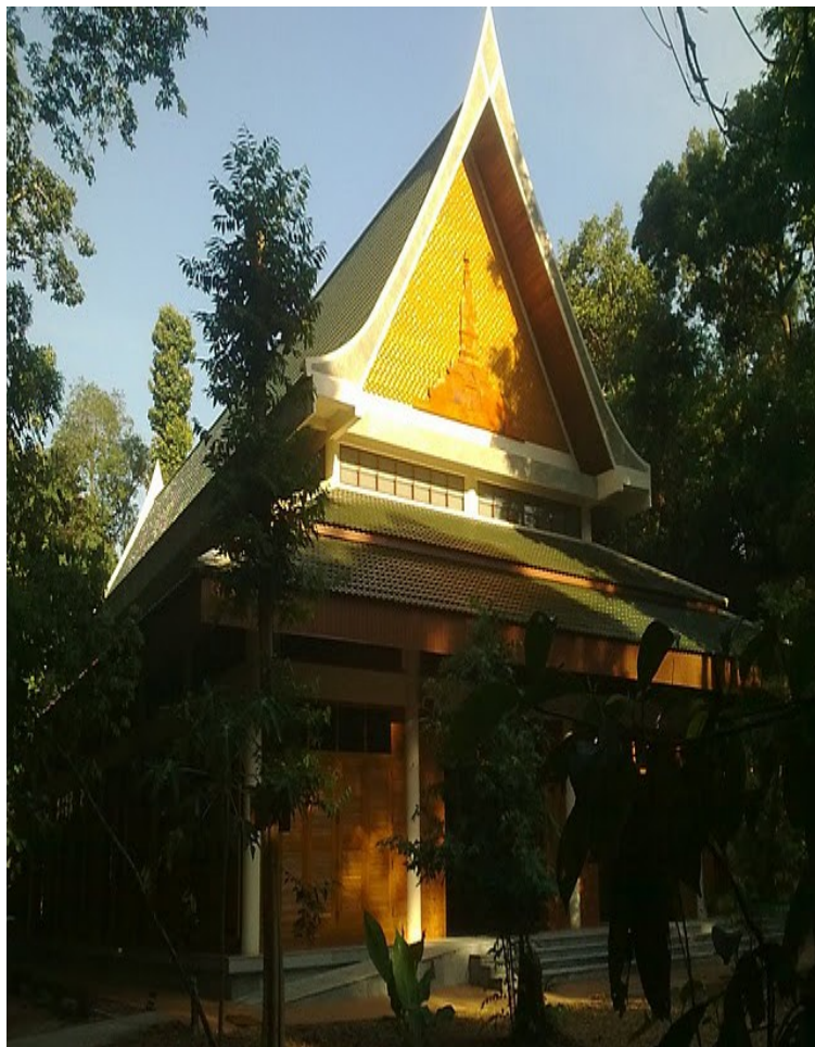
Above: The recently new Sala at Wat Pah Nanachat
